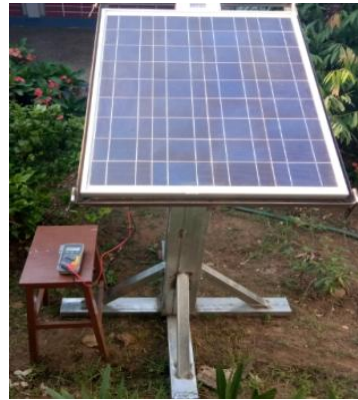
Figure 6. A solar PV panel without using reflector
