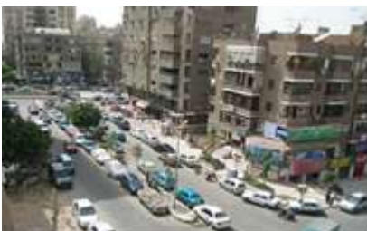
Fig. (28), Nasr City district, buildings have the same style. (Source: Authors)
