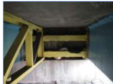
Connection of truss over main beam
