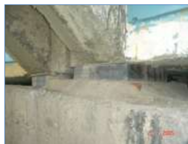
Replacement of damaged Bearings with new
