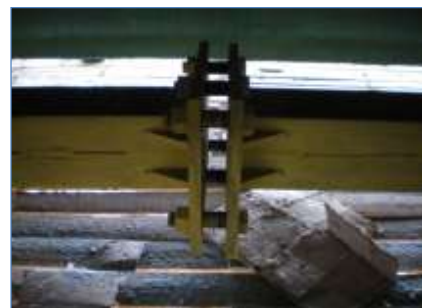
Pre-stressing Mechanism in Truss
