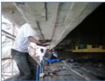
Groove for carbon Fibre composites laminates
